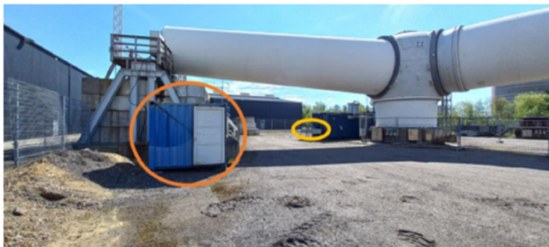
Overview of the blade test rig area as seen from West. Highlighting the two main noise sources which are the container with the hydraulic pump (brown) and the cooling fans (yellow).
